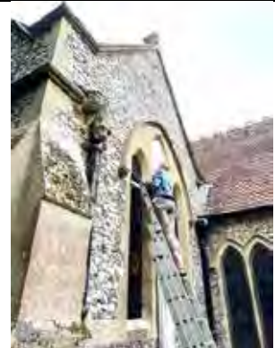
Figure 8 Installing the right-hand light (Ch.3)
